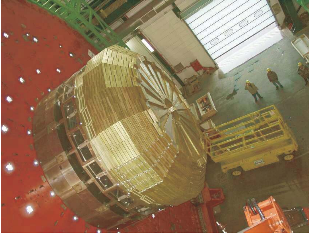
Figure 5.12: Partially assembled HE-minus absorber in the CMS surface hall (SX5). Scintillator trays can be seen to be inserted in some of the outer sectors.
